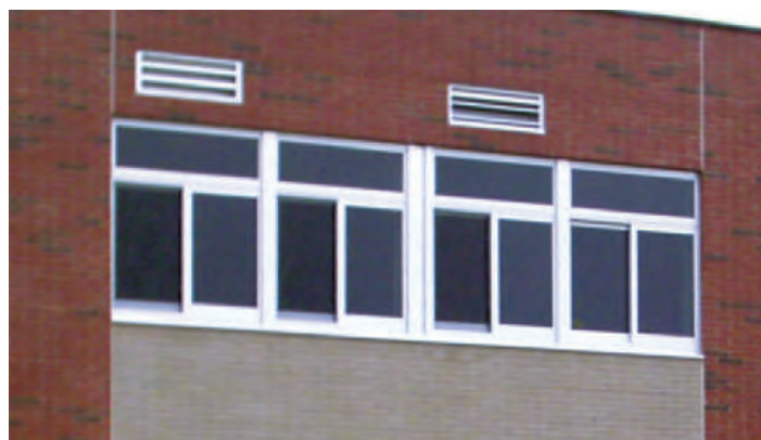
New Palz Central High School, New Palz, New York Architect: Collins & Scoville Architects, P.C. Glazing Contractor: Forno Enterprises, Inc. Systems Used: YES 45 FI, YES 45 TU, YSW 400 T & YVS 400 TU
