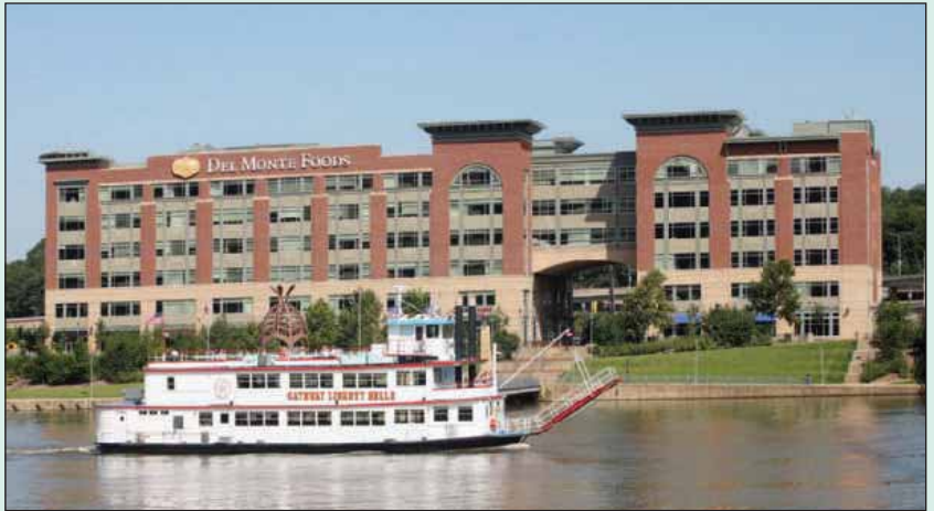
Del Monte Foods, Pittsburgh, PA Architect: Strada Architecture
